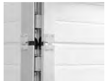
Detail of the concealed hinges of the pass door (inside view).
