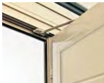
Detail of the opening limiter installed in the upper part of the leaf.
