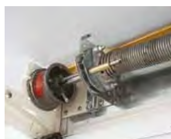
Cable break device that engages in the event of breakage of the springs that instantly stops the door operation (mandatory).
