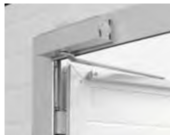
Detail of the overhead door closer mechanism of the pass door (inside view).
